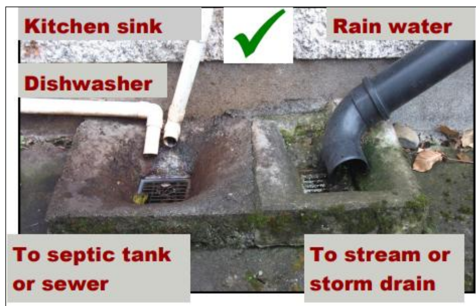
Figure 42. Correctly plumbed premises.
